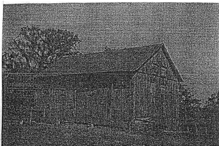
Unpainted building, made out of walnut wood, inside of which stage coach passengers alighted.
